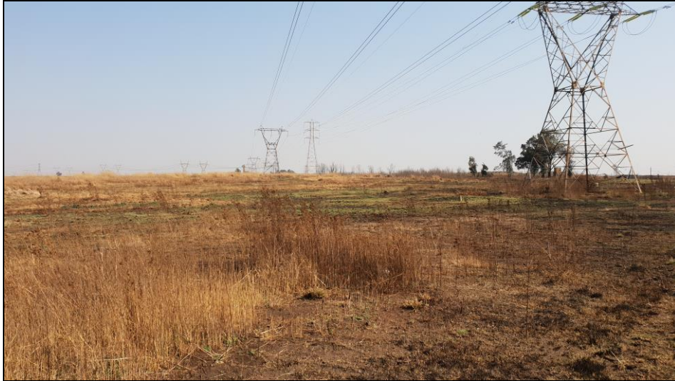
Figure 9: General view of existing infrastructure (power lines)
