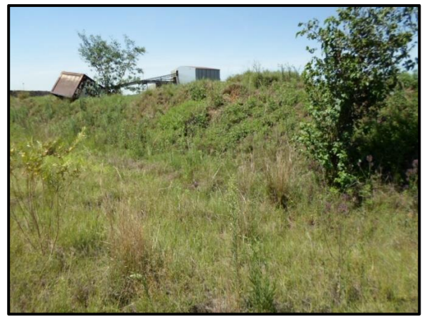
Figure 9. General site conditions
