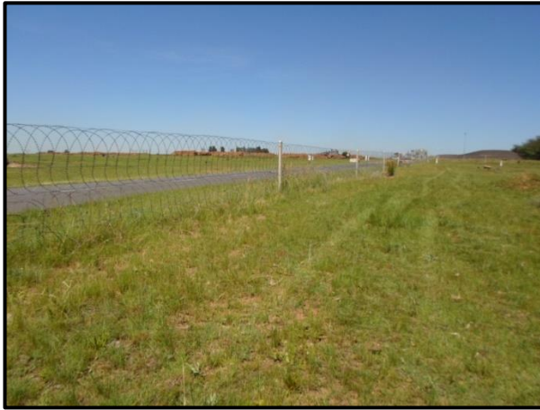
Figure 6. General site conditions
