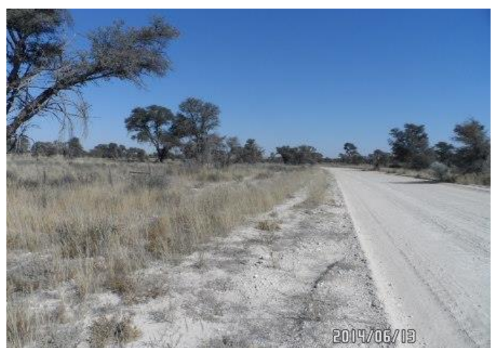
Photo 6: Looking west down R31
