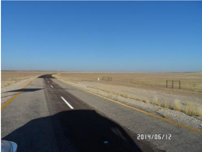
Photo 15: Looking east down R31 at Koo Pan. Pipeline will be located on southern side of the road (right of image).
