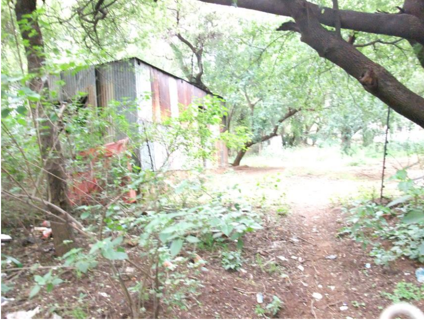
FIGURE 6: CORRUGATED IRON BUILDING IN THE SURVEYED AREA.
