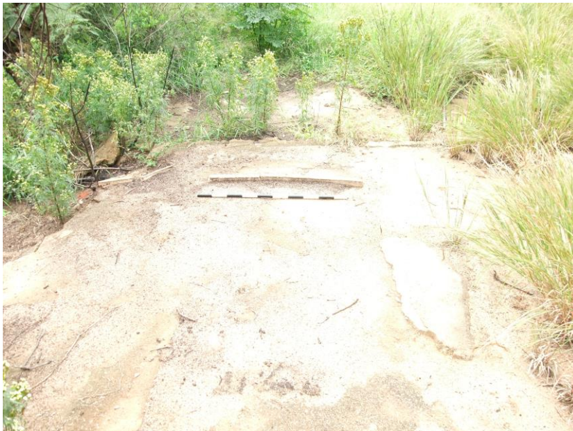
FIGURE 17: REMAINS OF ONE OF THE CONCRETE FLOORS.
