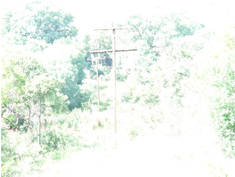
FIGURE 9: TELEPHONE LINES IN THE SYUDY AREA.
