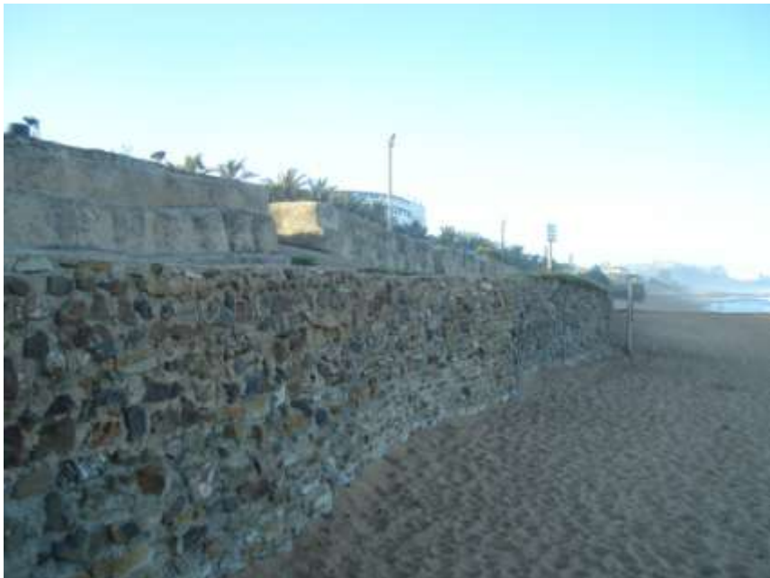
Existing sea wall
