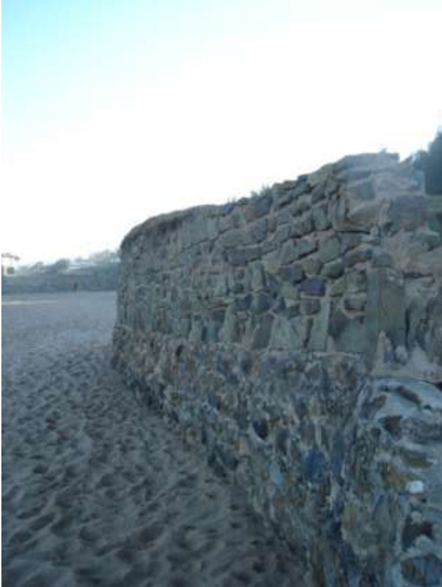
Existing sea wall
