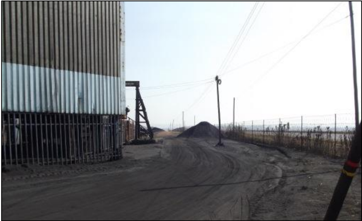
Fig. 5. Site KSO 3. The pipe will arrive at this loading station from the north-west.
