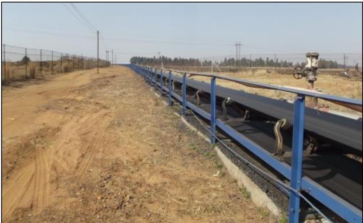
Fig. 4. Site KSO 2. Looking south-east. The pipe will run parallel to the conveyor belt system.
