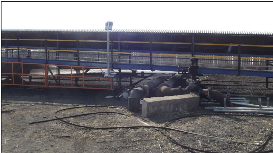
Fig. 2. Site KSO 1. Looking east. The pipe will come from this direction and then turn south.
