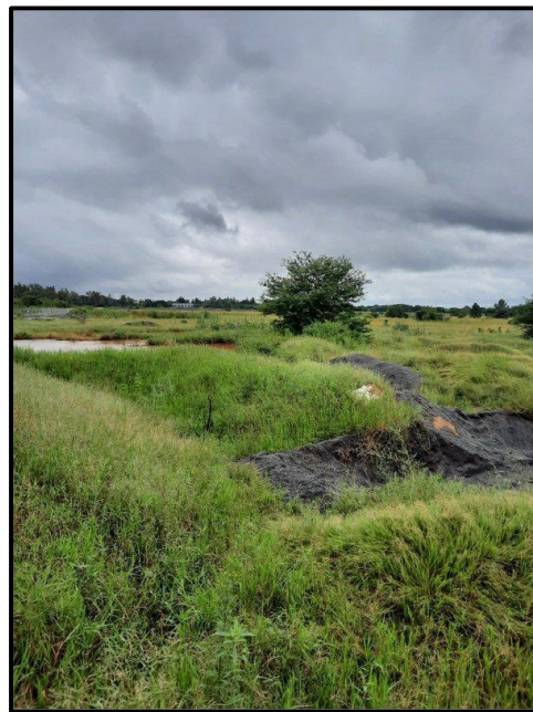
Figure 7.4. Earth moving activities evident throughout the area.
