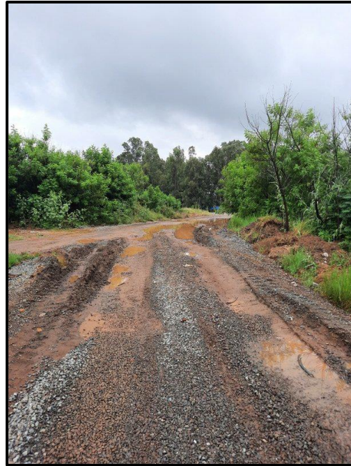
Figure 7.2. Main access road into the proposed project area.
