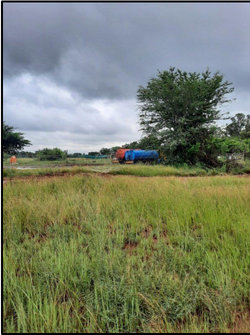
Figure 7.1. General site conditions showing the existing site office.
