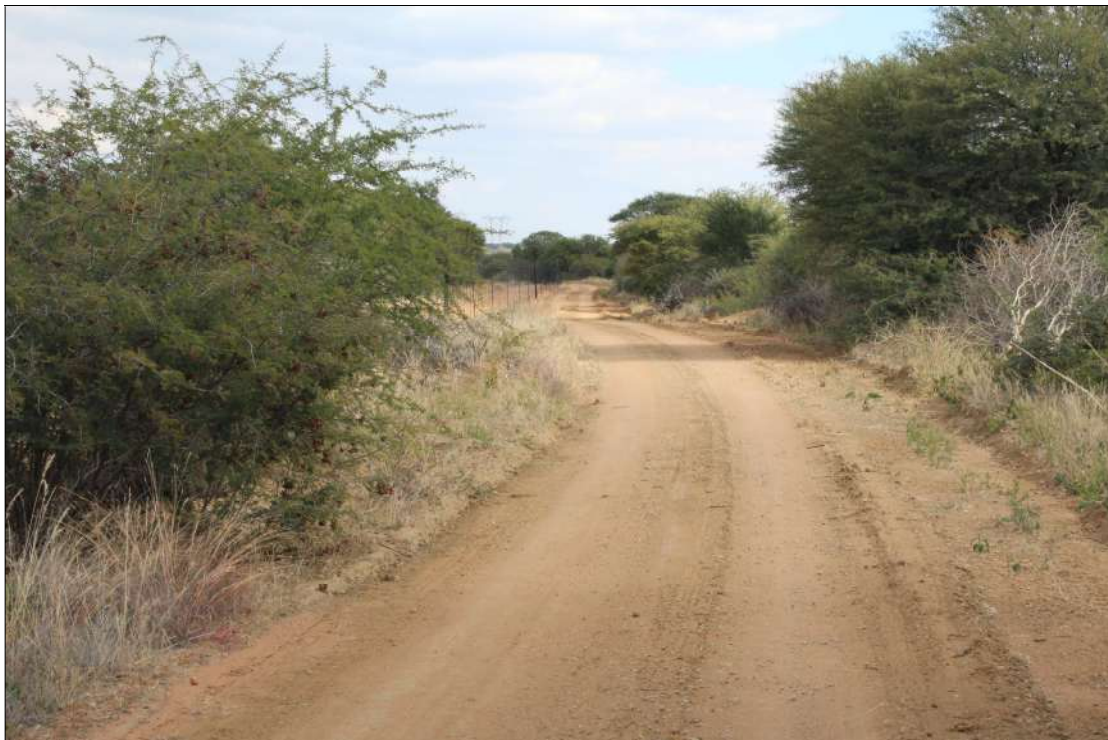
Figure 4: Access gravel road alongside the rail tracks
