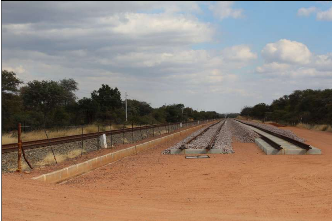
Figure 1: Existing Railway tracks
