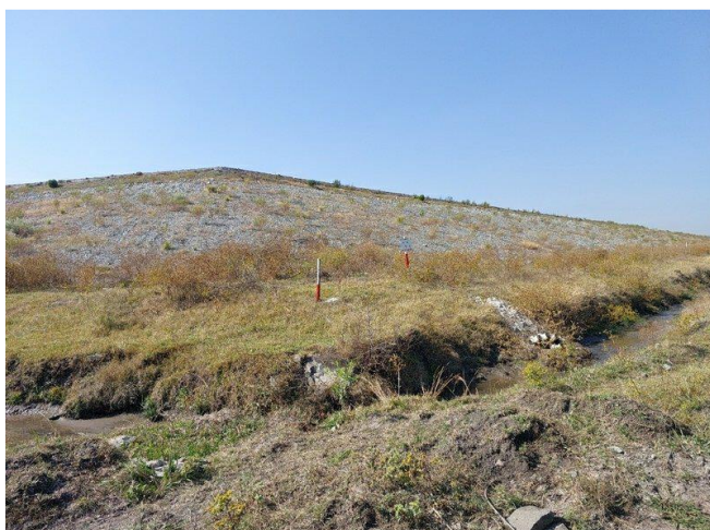
Figure 5.3. General site conditions viewed from the east.
