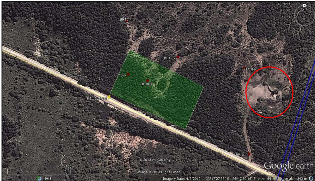
Figure 40. Close-up aerial view of the area proposed for Borrow Pit 10 (BP10) showing the plotted general GPS points and existing diggings (red circle).
