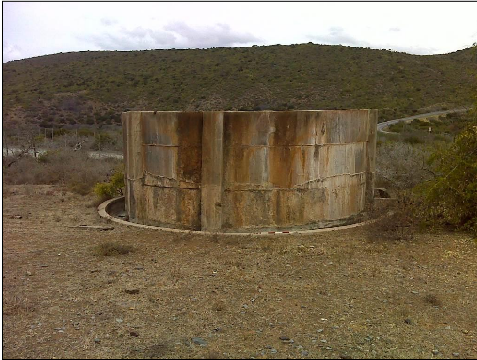
Figure 16. View of the disused water reservoir situated outside of the area proposed for the borrow pit.
