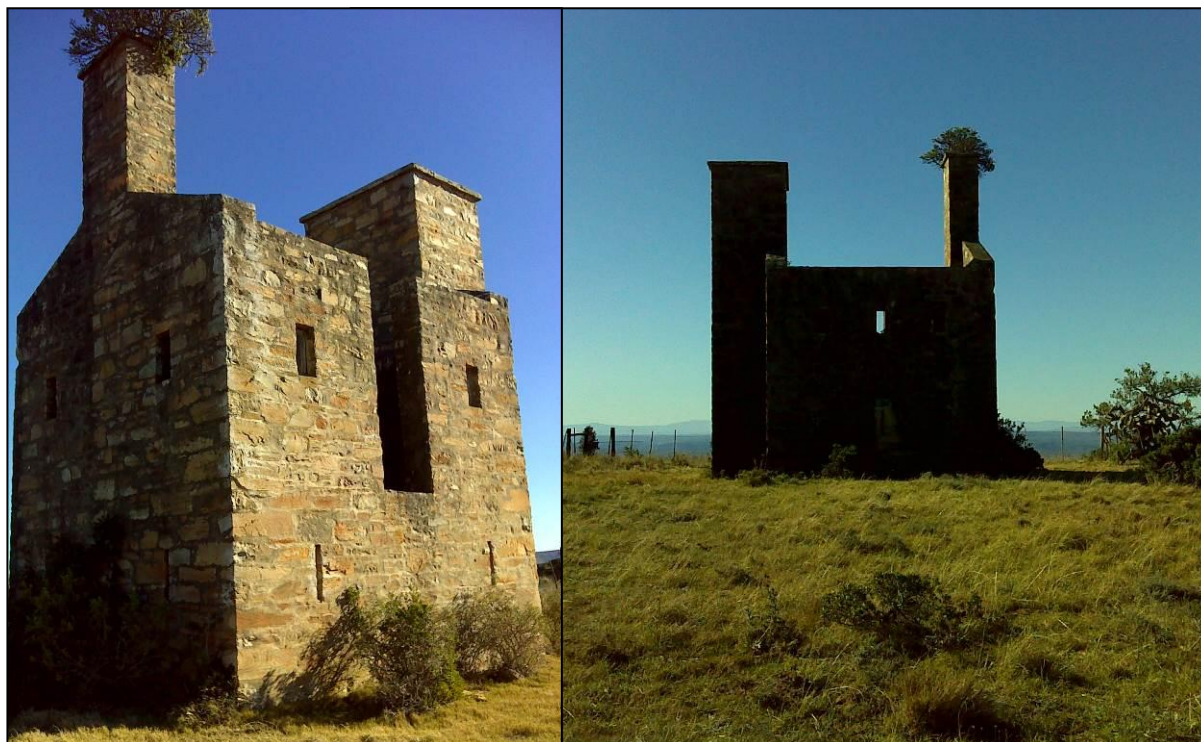
Figure 74. Alternative views of the Fraser's Camp Signal Tower.
