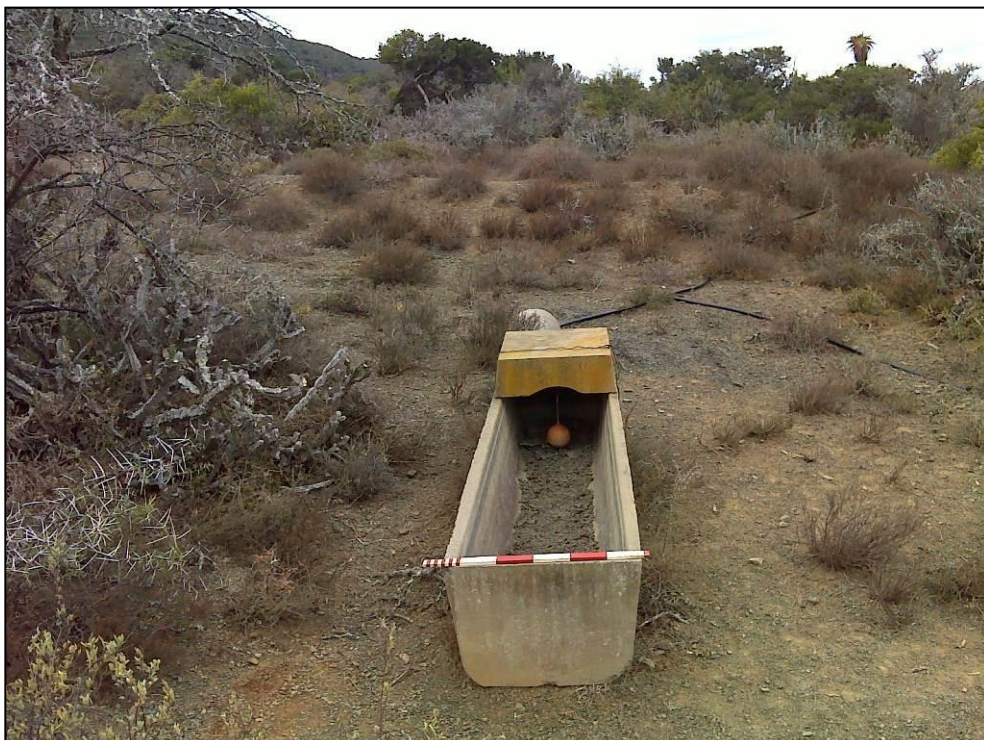
Figure 17. View of the disused water trough situated outside of the area proposed for the borrow pit.
