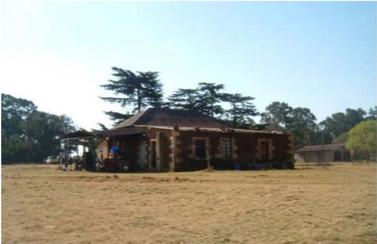
Figure 28 - HH05 was constructed with sandstone and ferricrete. It was extended with a lean-to which was also built with ferricrete whilst the corner posts of the structure were decorated with blocks of sandstone. The residence was built in the early 19 th century (above).
