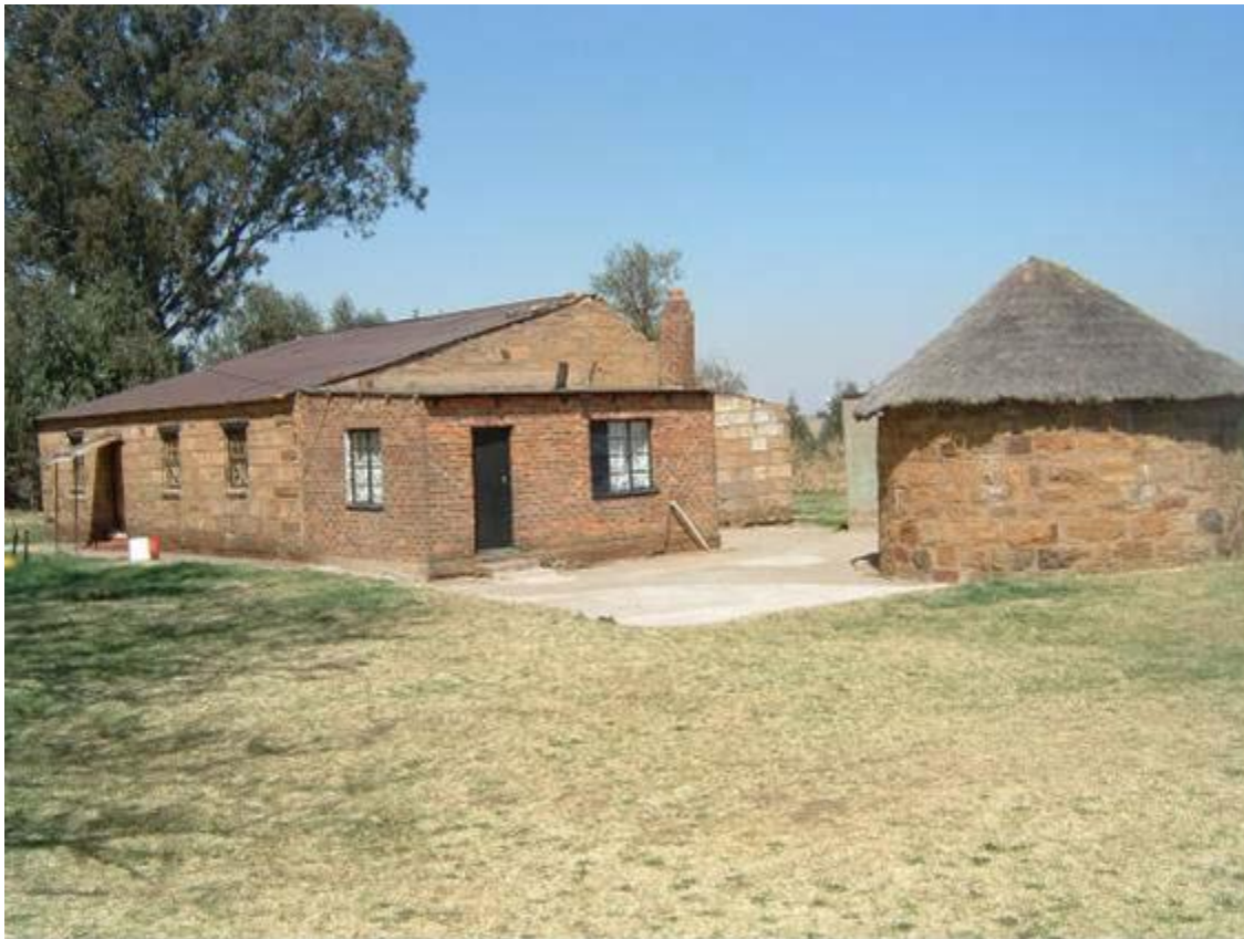
Figure 15 - FC02 on the farm Grootlaagte 449JS is composed of a house and rondavel constructed with sandstone. A dilapidated ferricrete structure, with probably served as a wagon shed, is part of this complex (above).
