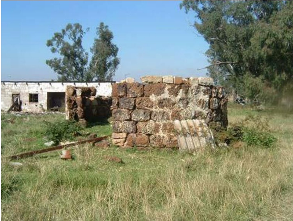
Figure 32 - A rondavel which was constructed with ferricrete is part of FC08 on the farm Schoonoord 164IS. It was probably fitted with a pitched corrugated iron roof (above).
