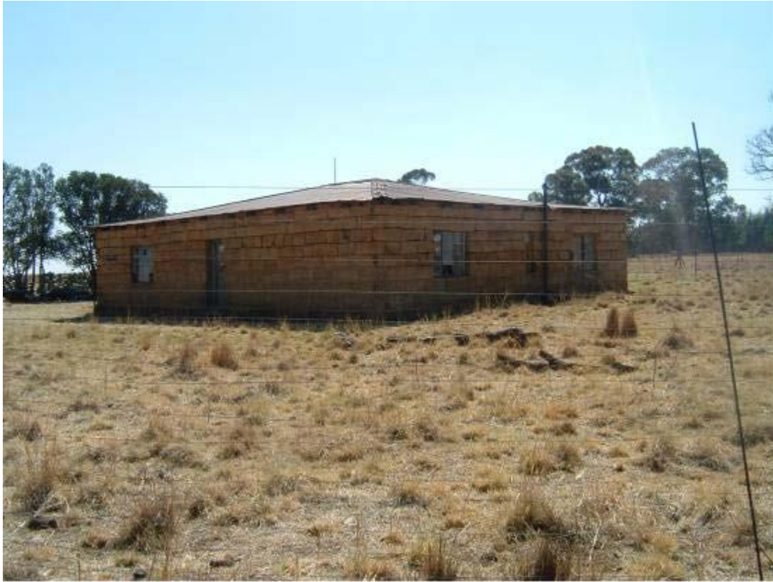
Figure 18 - HH02 is a square house which was constructed with sandstone on the farm Grootlaagte 449JS (above).
