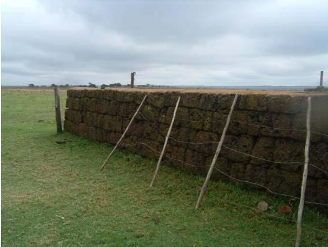
Figure 7 - A cattle enclosure (CE02) on Portion 06 of the farm Mooifontein 448JS constructed with ferricrete. It is highly likely that this structure was associated with a farmstead complex which was constructed with identical building material and with sandstone (above). The farmstead complex to which the cattle enclosure belonged may have been demolished in the past.
