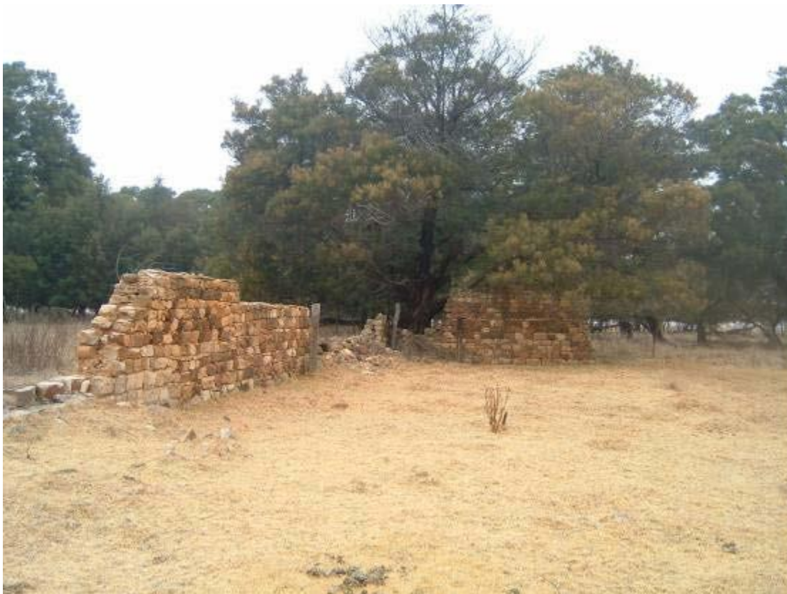
Figure 4 - The remains of a possible residence and wagon shed on the farm Mooifontein 448JS which were linked with each other in more recent times to be used as a cattle enclosure (above).
