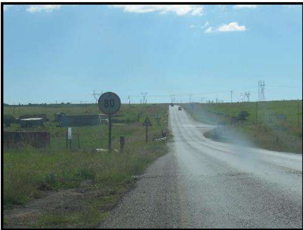
Figure 5. Section of the proposed pipeline trajectory between Hattingspruit and Dannhauser. None of the existing homesteads adjacent to the road contains any graves.
