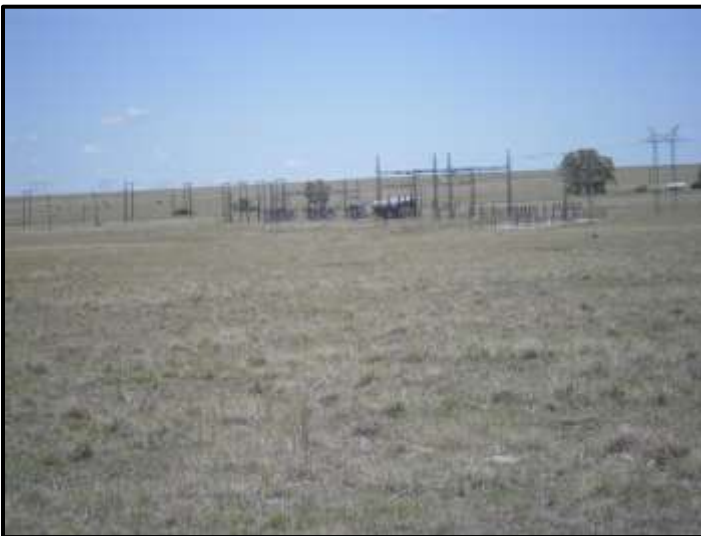
Figure 9. Substation that power will feed into.
