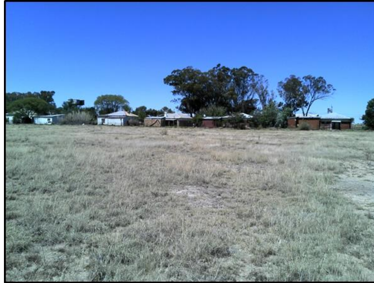
Figure 12: Plessis Railway station houses viewed from PV1
