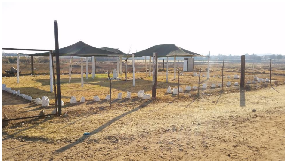
Figure 10: General view of the temporary structures in the southern section of the survey footprint
