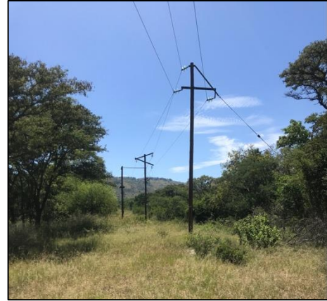
Figure 21 – View of existing powerlines.
