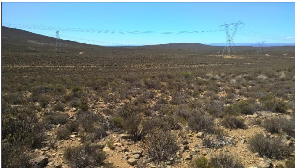
Figure 6: View of the area proposed for substation alternative SS1 facing north (Fortuin 74).
