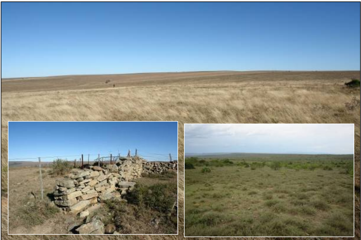
Fig. 4. General views of the proposed southern powerline route from the Kopleegte Substation towards the proposed Golden Valley Substations and the dry packed stone wall close to the route.
