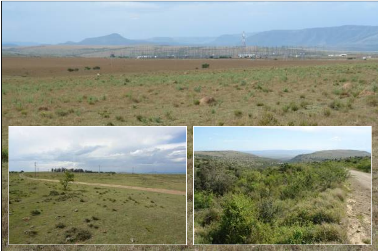
Fig. 1. The Poseidon Substation (main image) and views of the flat plateau the green powerline follows before it descends down the steep escarpment into the Great Fish River Valley (right insert).
