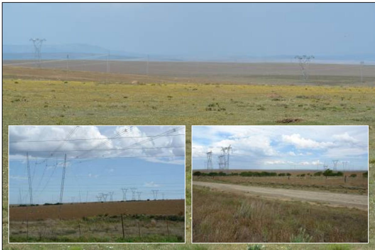
Fig. 2. General views from the Poseidon Substation towards the proposed Golden Valley Substations (main image) and the existing power lines routes which the proposed middle and eastern power lines follow.
