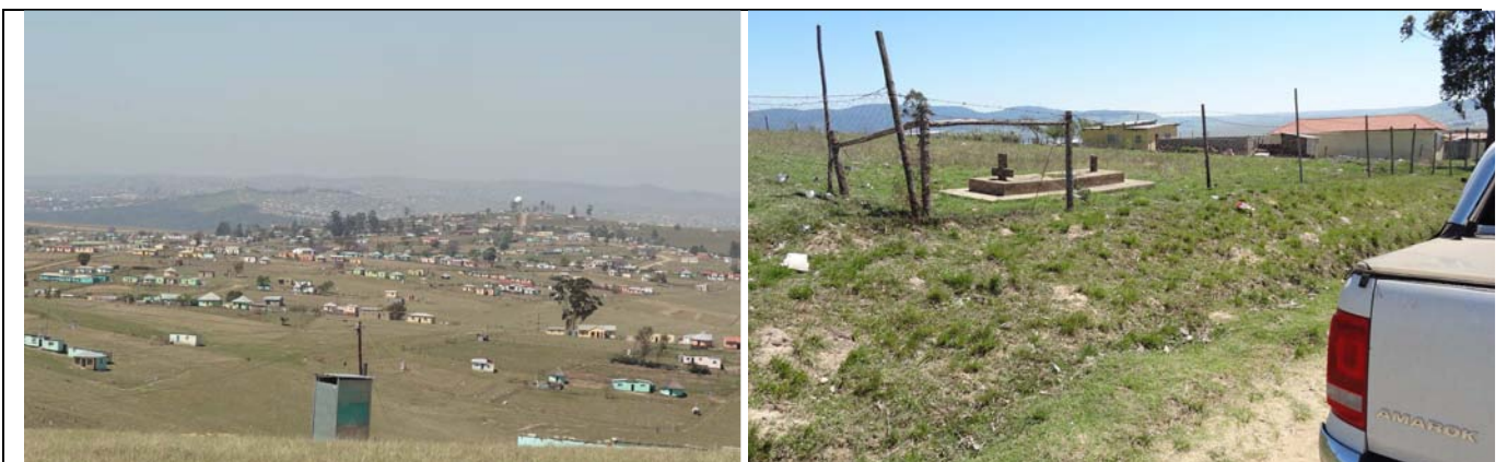
Plate 5: Photo 9 and 10 shows some of the built up areas along the Nqadu (Mavete-Lower Gungululu bulk water pipeline route) and a burial site barely 10m from the proposed Nqadu (Mavete-Lower Gungululu) pipeline servitude (Author 2013).
