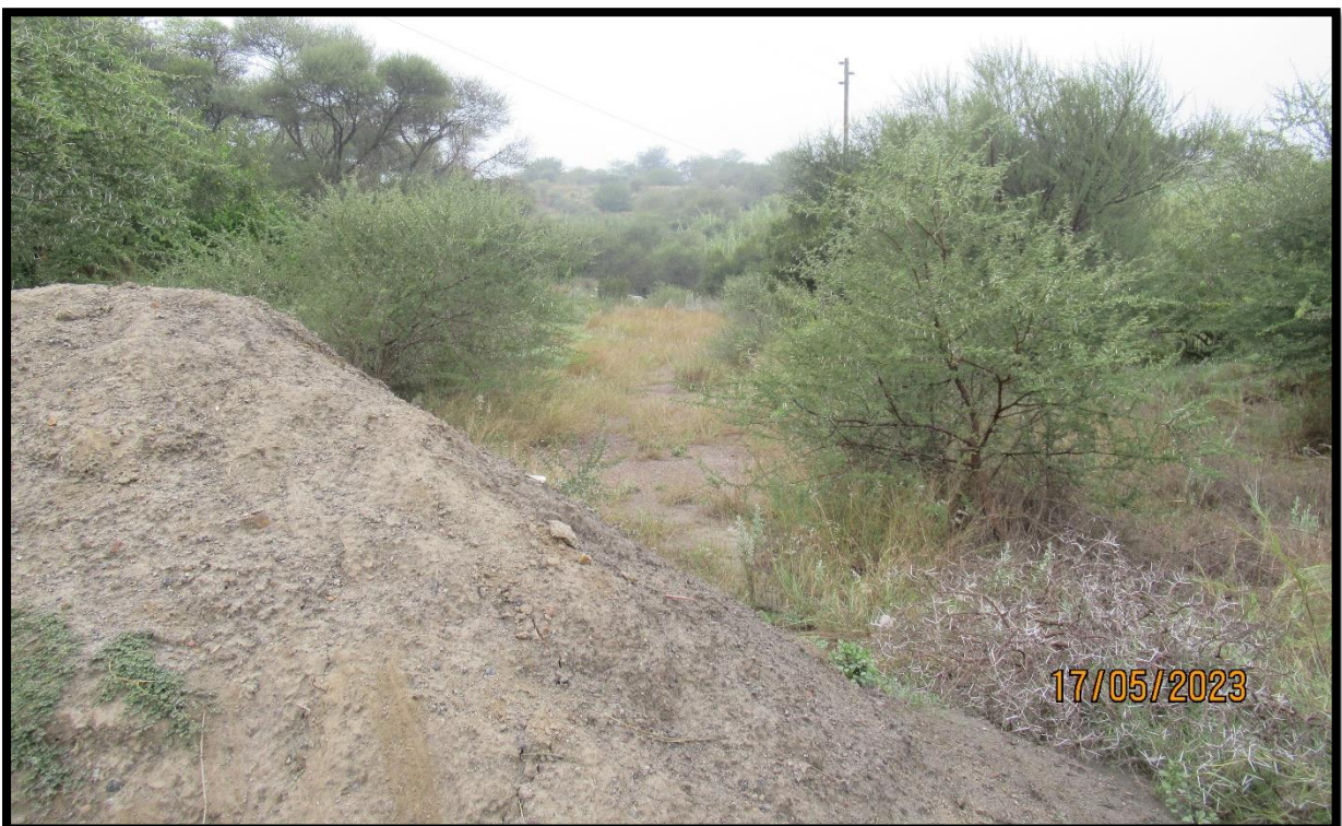
Figure 8: View in north-west near corner. Berm visible.
