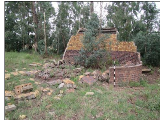
Figure 36 – b) Brick silo at LES011
