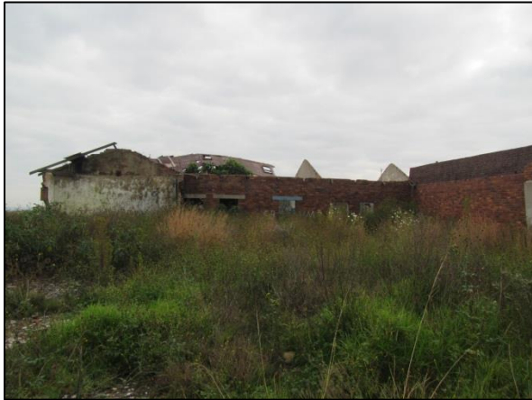
Figure 23 – Front view of brick structure at LES004
