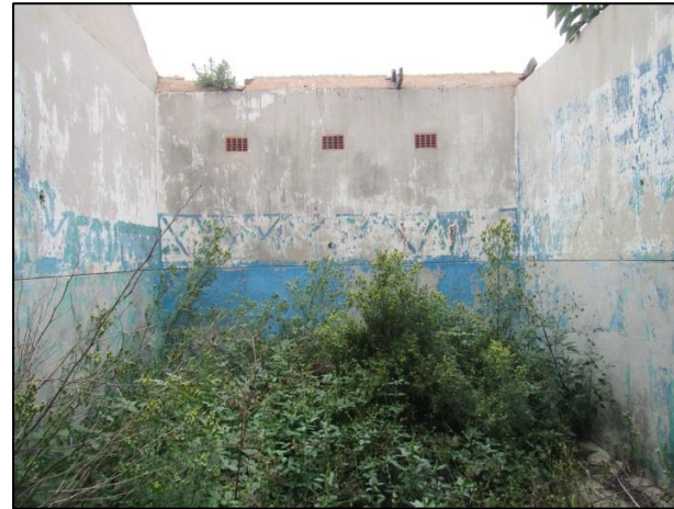
Figure 26 – Painted room LES004
