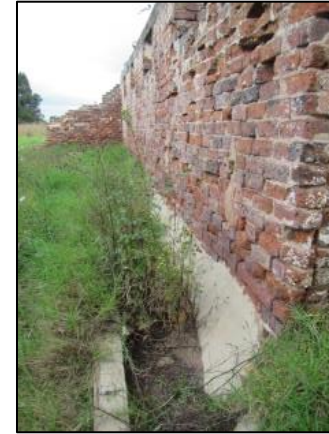
Figure 41 – Concrete trough within stable at LES012
