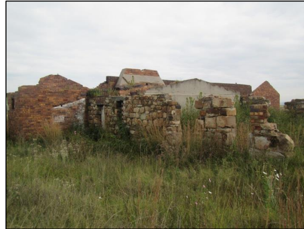
Figure 24 –Rear view of structure with stone-built addition at LES004
