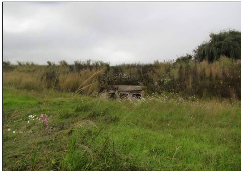
Figure 68 – Old culvert at LES026
