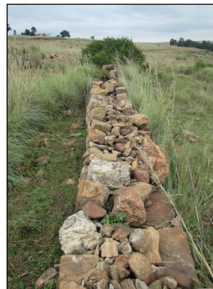
Figure 64 – Detailed view of stone wall at LES023
