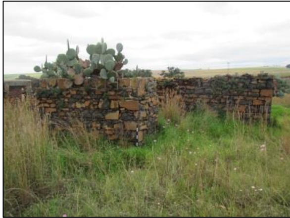
Figure 42 – b) Stone-and-brick structure at LES012
