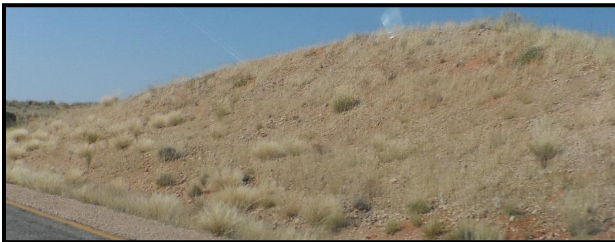
Photo 28: Calcrete used to stabilize steeper slopes of dunes within the existing road reserve
