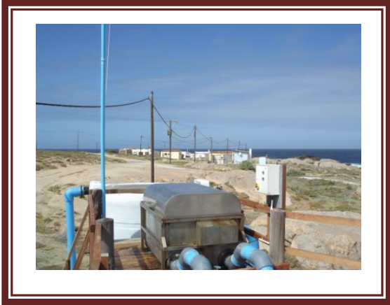
Ou Lokasie seen from Storage tanks looking south
