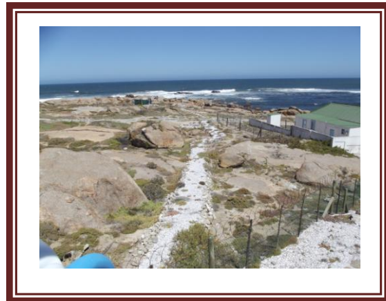
View towards sea showing present inlet pipe.
