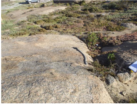
Site 7. Remains of cement channel on rock to channel rainwater into a catchment pond shown below, now silted up. The pond was used by the residents of Ou Lokasie to wash with.
