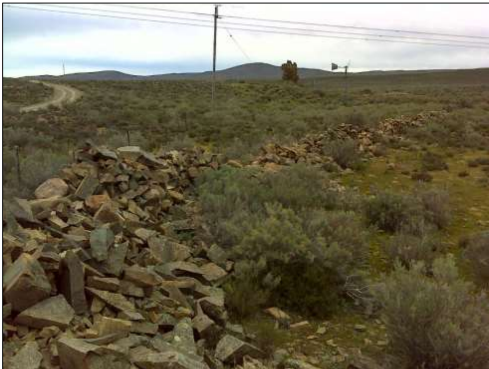
Figure 20. View of the dry packed stone wall (K-PLSW2) on the Farm Standvastigheid 210.
