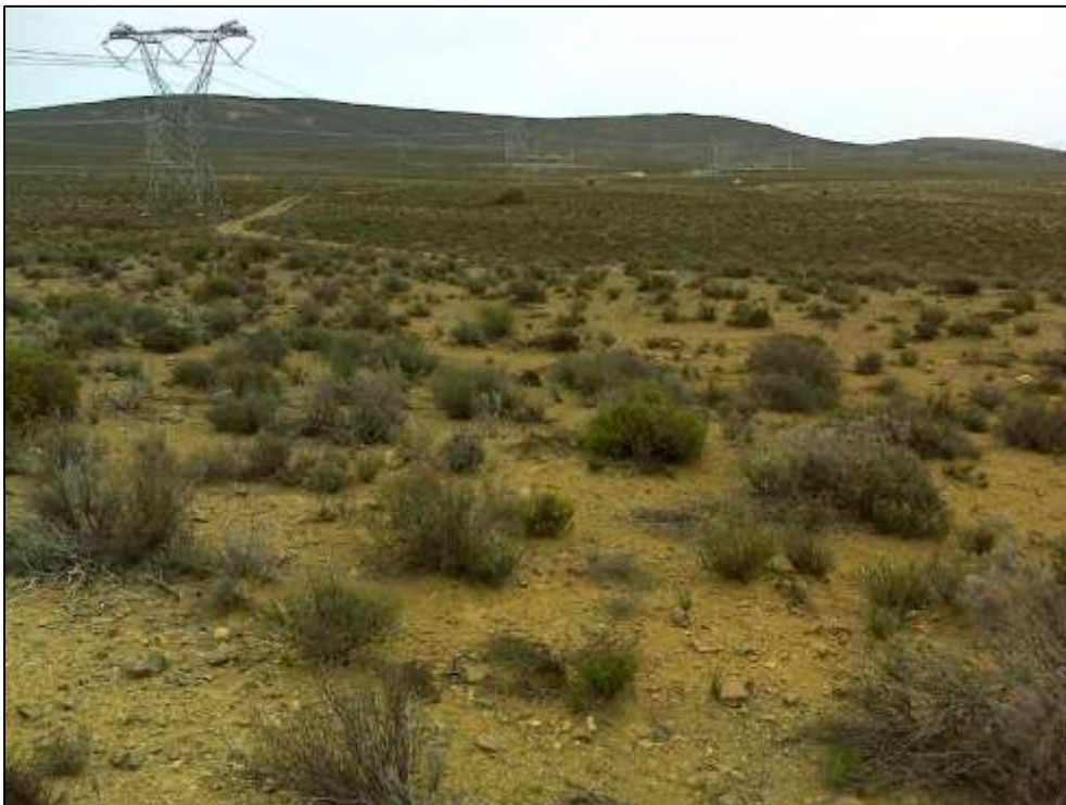
Figure 8. General landscape of the power line route on the Farm Standvastigheid 210.
