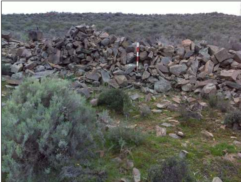
Figure 19. View of the dry packed stone wall (K-PLSW2) on the Farm Standvastigheid 210.
