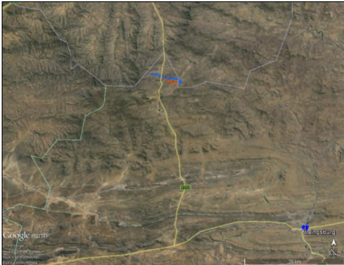
Figure 1: The powerline crosses the R354, some 20km north of Matjiesfontein on the road to Sutherland.
