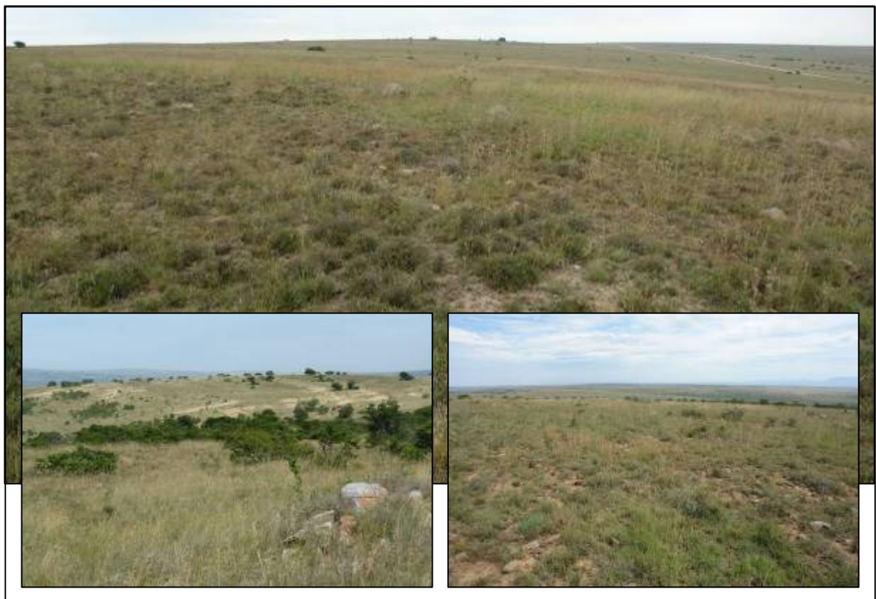
Figure 9. Views of the turbine positions 14-24 (main image), 45-18 (left insert) and 37-47 (right insert).
