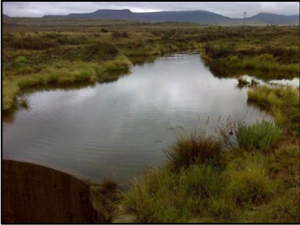
Figure 6. View of the large donga and associated weir infrastructure.
