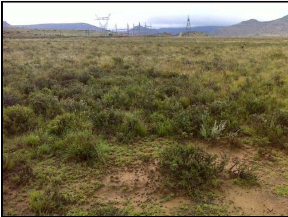
Figure 7. View of the landscape and the existing substation in the distance.
