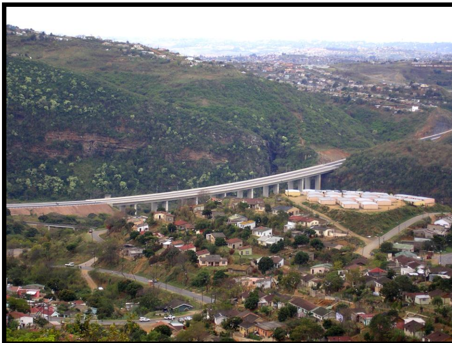
Figure 5. Photograph showing the section of the proposed trunk road development crossing the Umgeni River. No heritage sites were located in the near vicinity of the road development.
