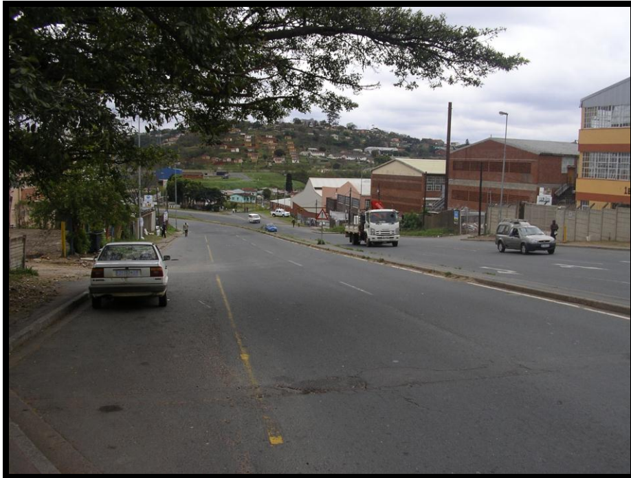
Figure 2. Section of the proposed trunk route linking the CBD of Pinetown with Clermont.
