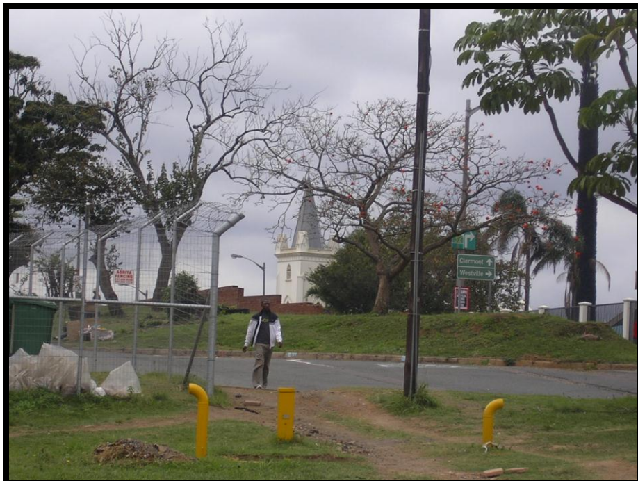
Figure 3. Although historical buildings occur in Pinetown none of them occur closer than 30m from the proposed C3 Trunk Road development. An old church building is seen in the distance.
