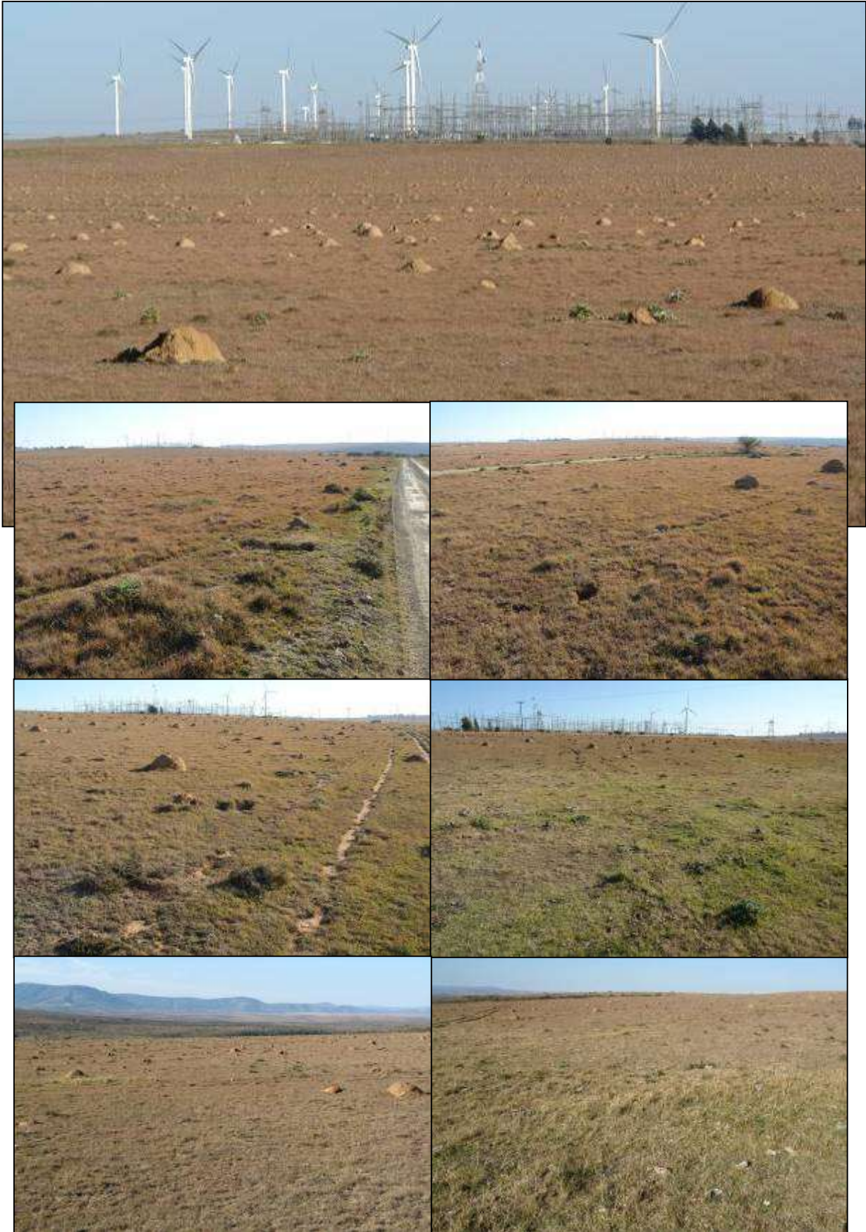
Figure 1. General views of the proposed area for the construction of a facility substation complex, metering station and a 2 kilometre overhead power line to the Poseidon Substation.
