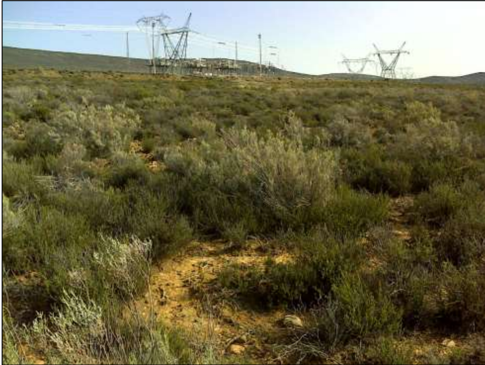
Figure 5. View of the general landscape of the proposed area of the existing Komsberg Substation facing south west with the existing substation and power lines in the background.
