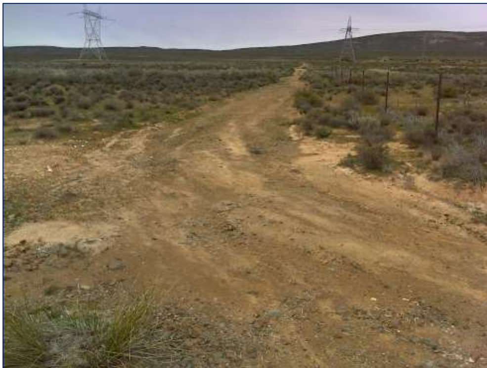
Figure 10. View of the access road to be widened facing east.
