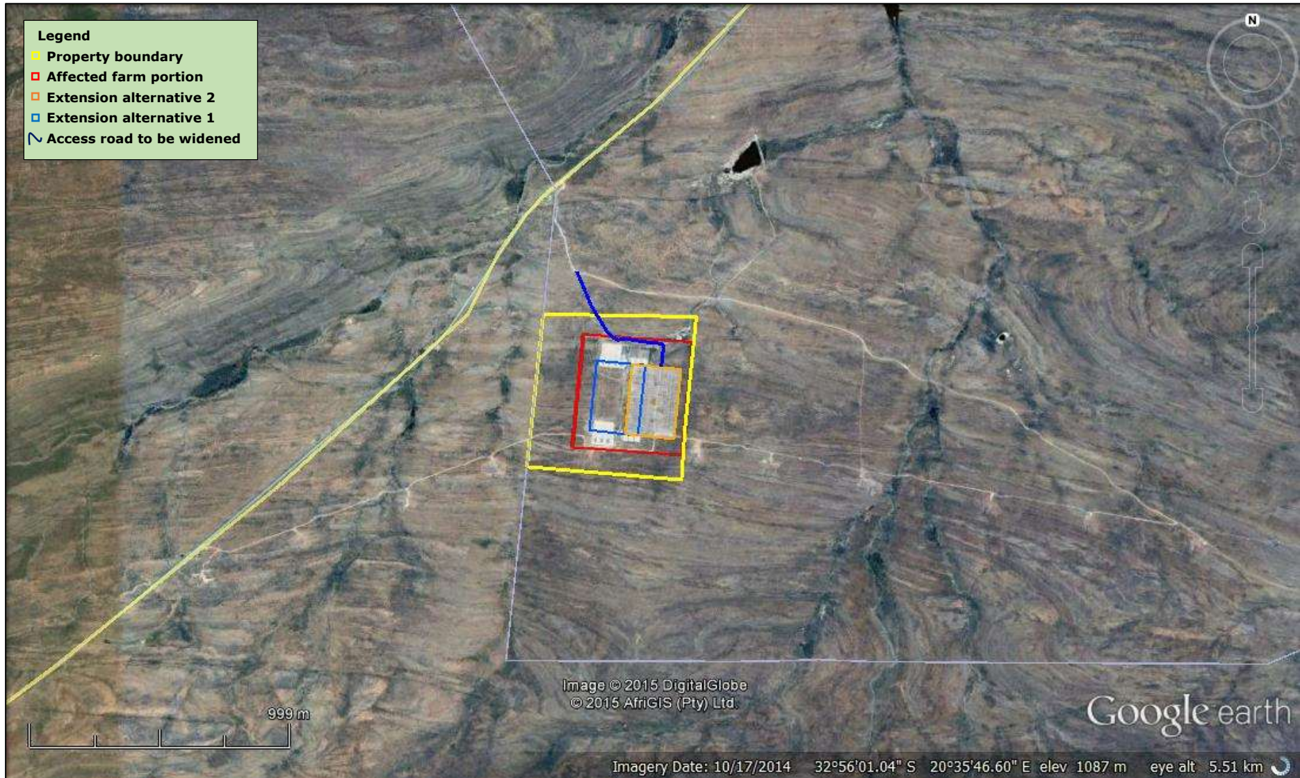
Figure 3. Aerial view showing the location of the proposed extension of the existing Komsberg Substation (two alternative areas) and widening of the access road situated on Eskom owned land on the farm Standvastigheid 210.
