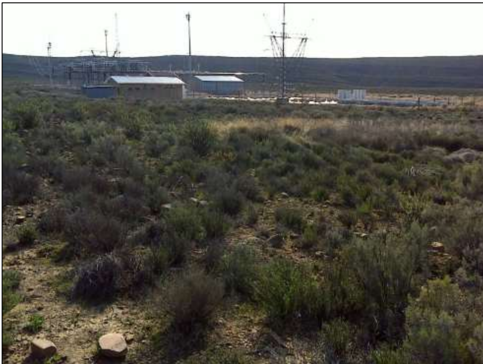
Figure 6. View of the general landscape of the proposed area of the existing Komsberg Substation facing north west with the existing substation and power lines in the background.
