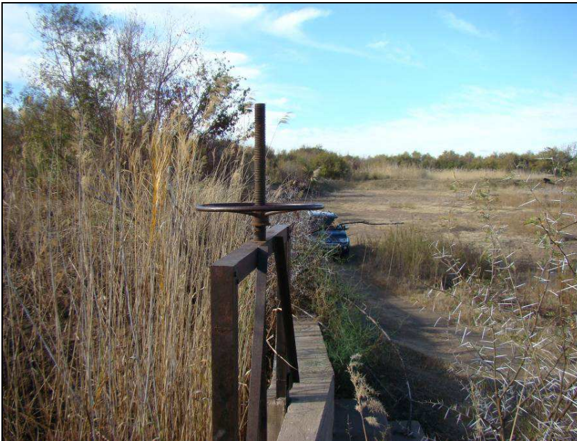
Fig.16 Floodwater control sluice at Soverby. Date 6/10/1989 inscribed in concrete.
