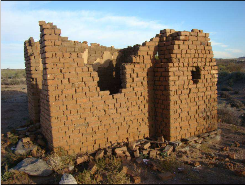
Fig.4 Ruin with bricks & mortar walls BP1 Soverby.
