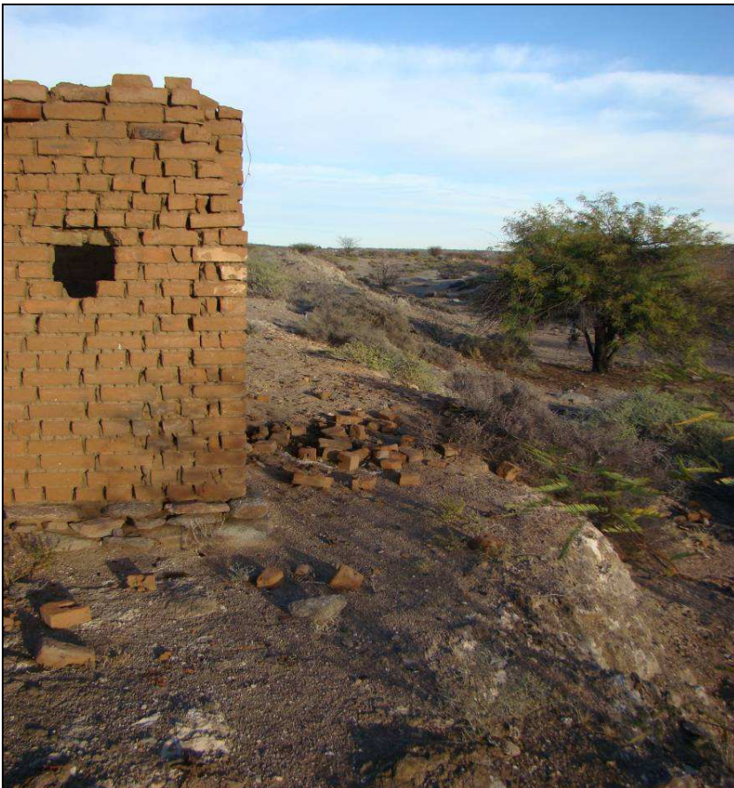
Fig.5. Ruin with bricks & mortar walls BP1 Soverby.
