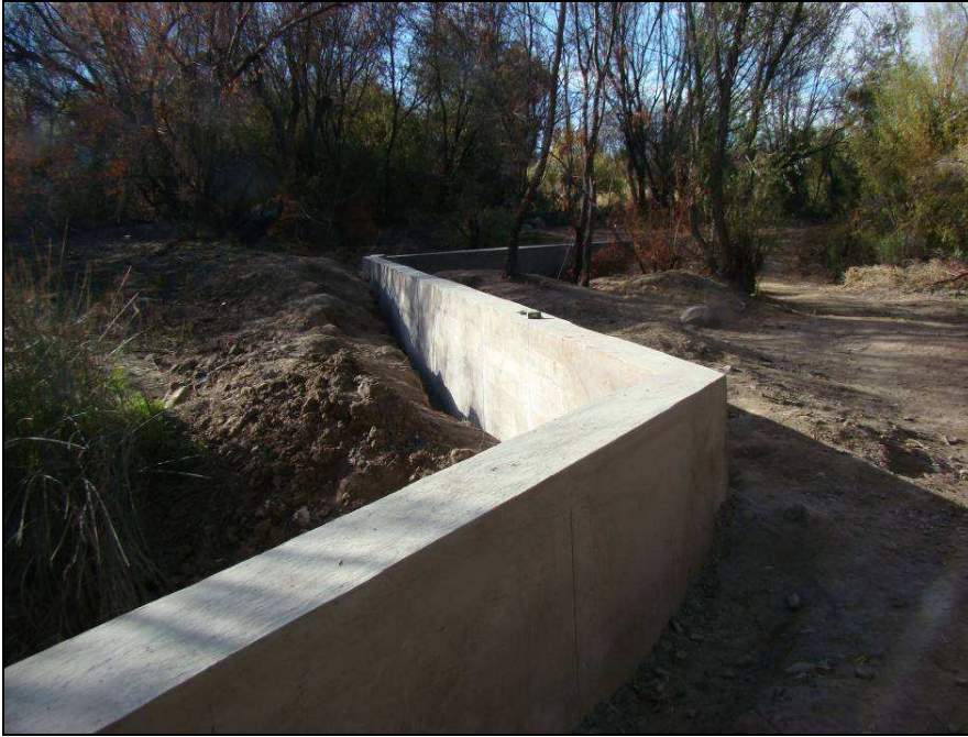
Fig.15 New weir in river branch at Soverby.
