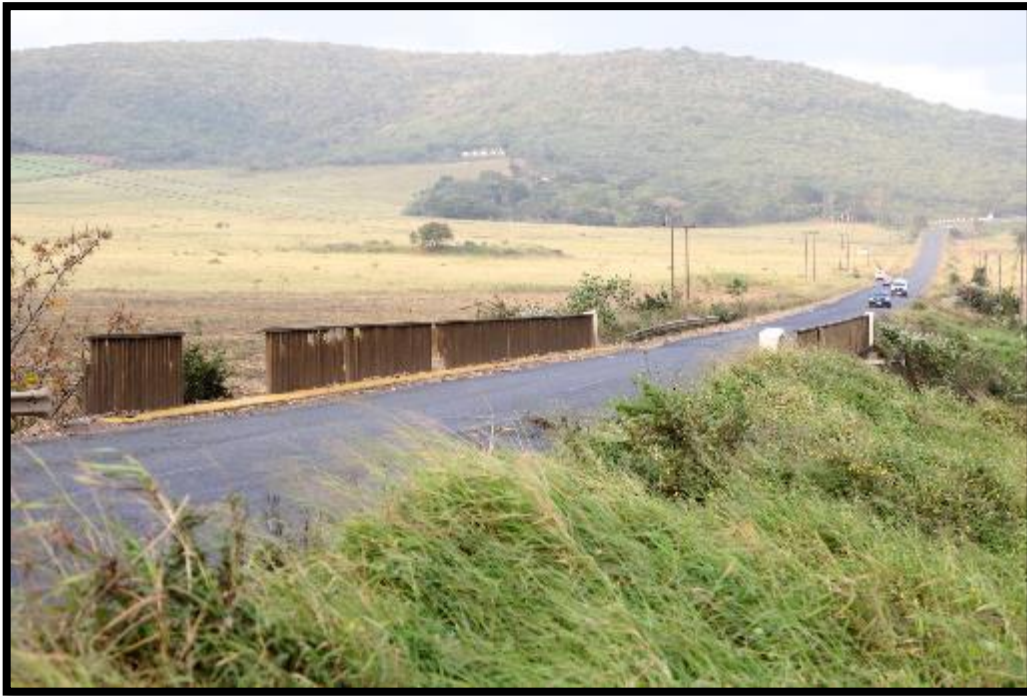
Figure 7: The P393 (R34) in the vicinity of the Dango Bridge.
