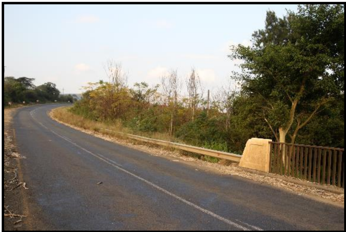
Figure 4: The P394 (R34) crossing the Bedlane Bridge.
