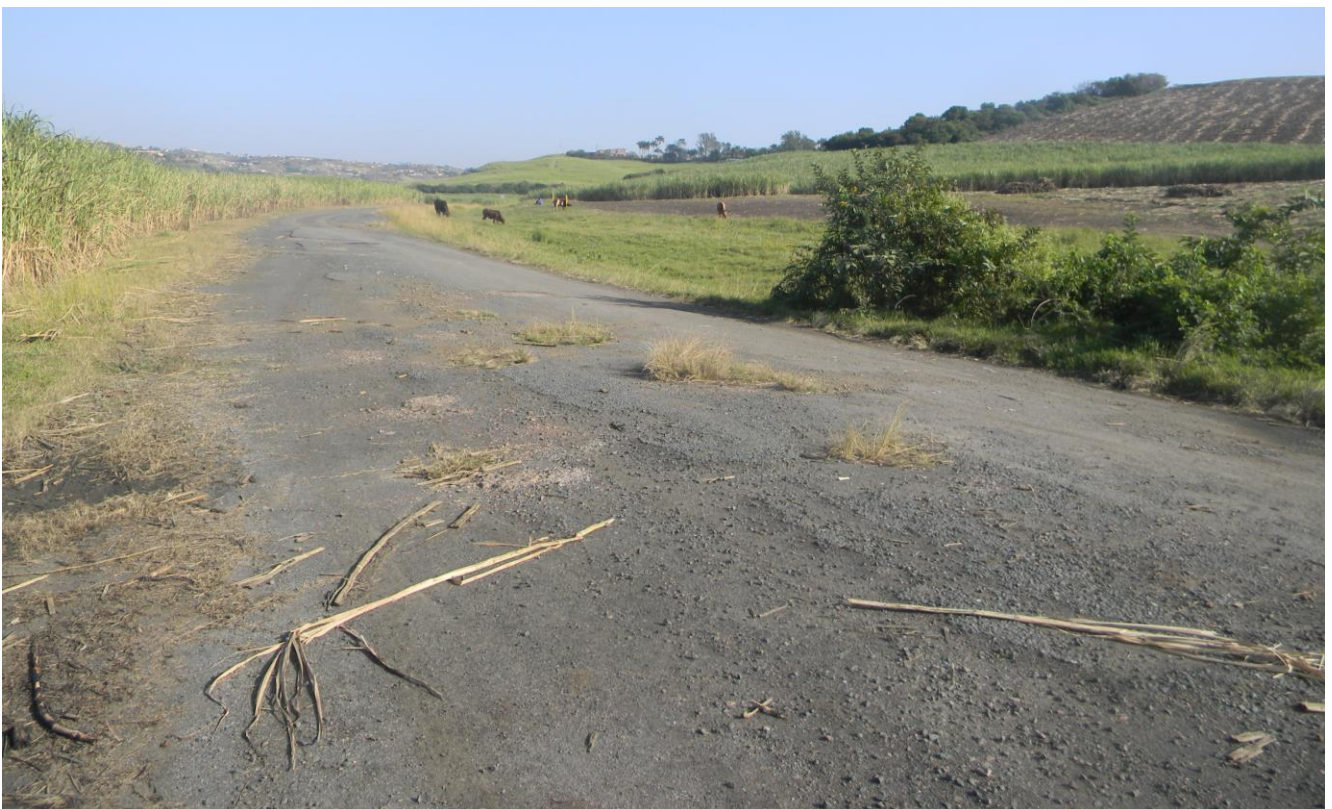
Plate 2: Photo 2: View of proposed pipeline route (Photograph © by Author 2019)
