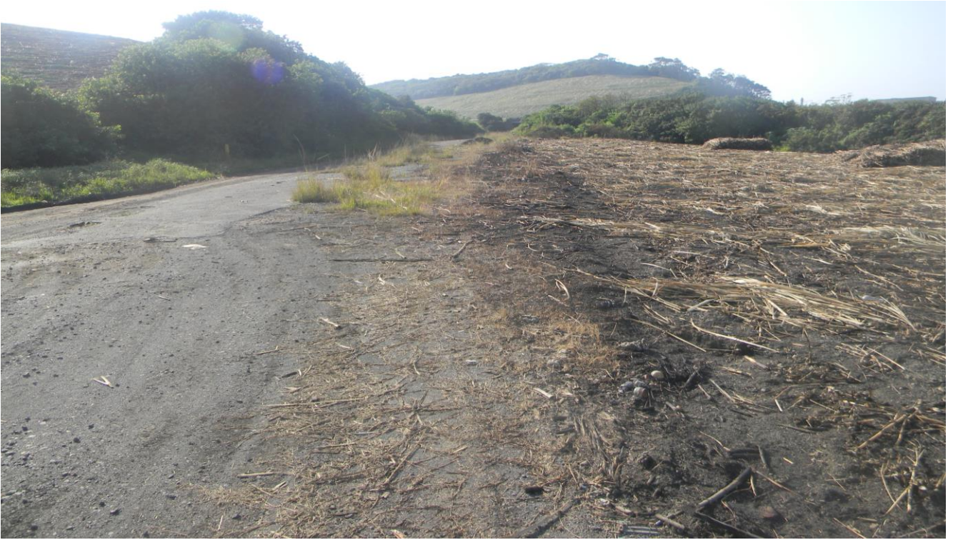
Plate 5: Photo 5: View of proposed pipeline route (Photograph © by Author 2019)
