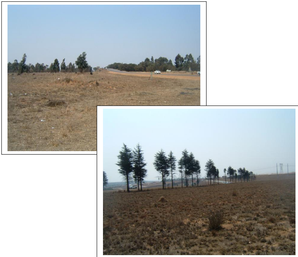
Figures 3 & 4- The northern stretch for the proposed deviation of Road 575 occurs in close proximity of a bridge which will be widened as part of the road deviation project (above and below).
