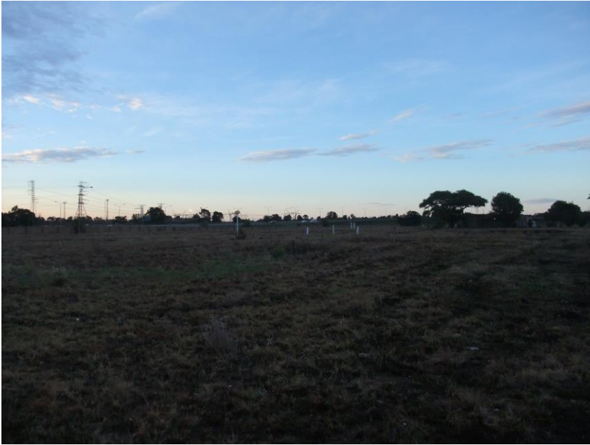
Figure 28: Here the pipeline runs together with power lines in a landscaped environment.
