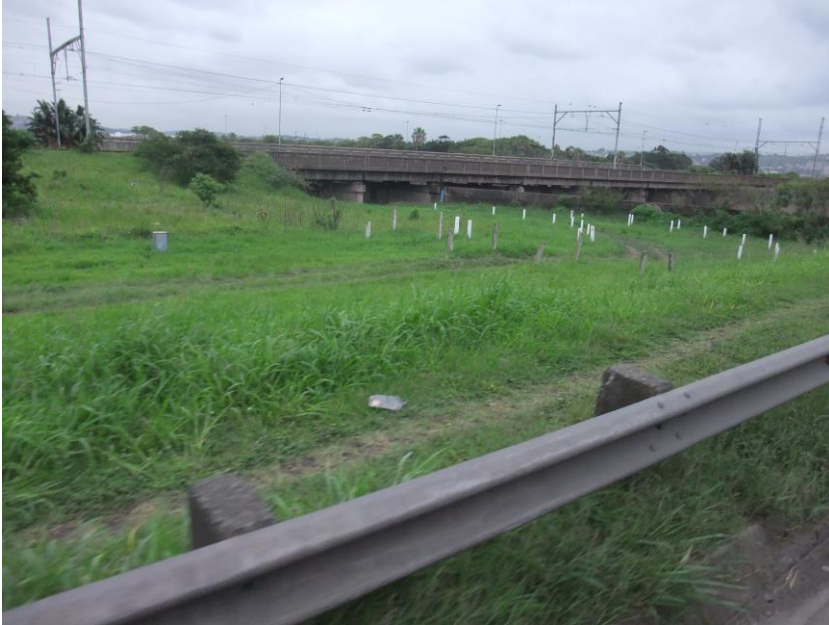
Figure 63: The pipeline in the Durban harbor area.
