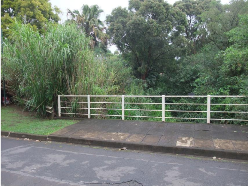
Figure 53: River crossing in Pietermaritzburg, where the pipeline is situated.
