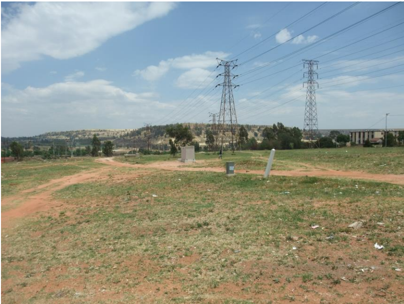
Figure 23: Here the pipeline runs together with power lines. Also note the mine dump in the background.
