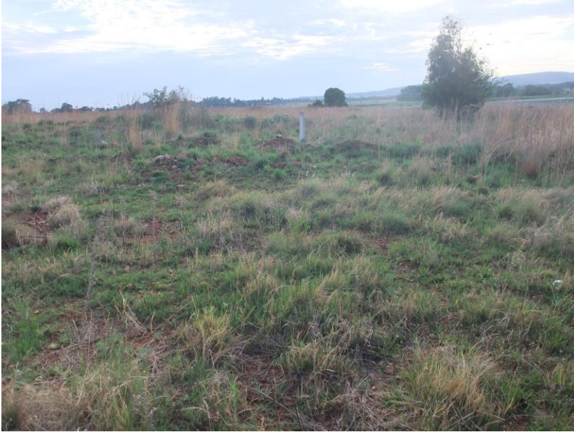
Figure 29: Earthwork activities along the pipeline route.
