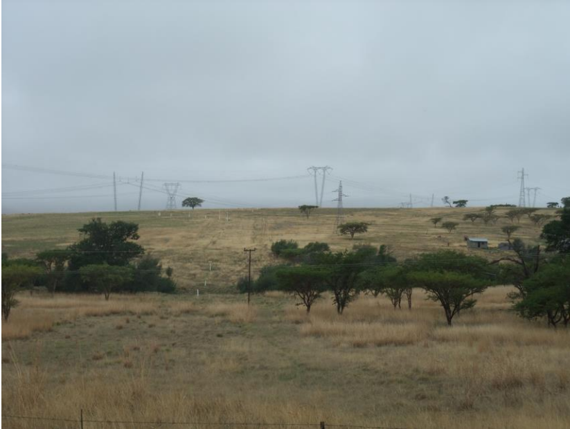
Figure 45: Note the pipeline servitude across rolling hills and adjacent to power lines.
