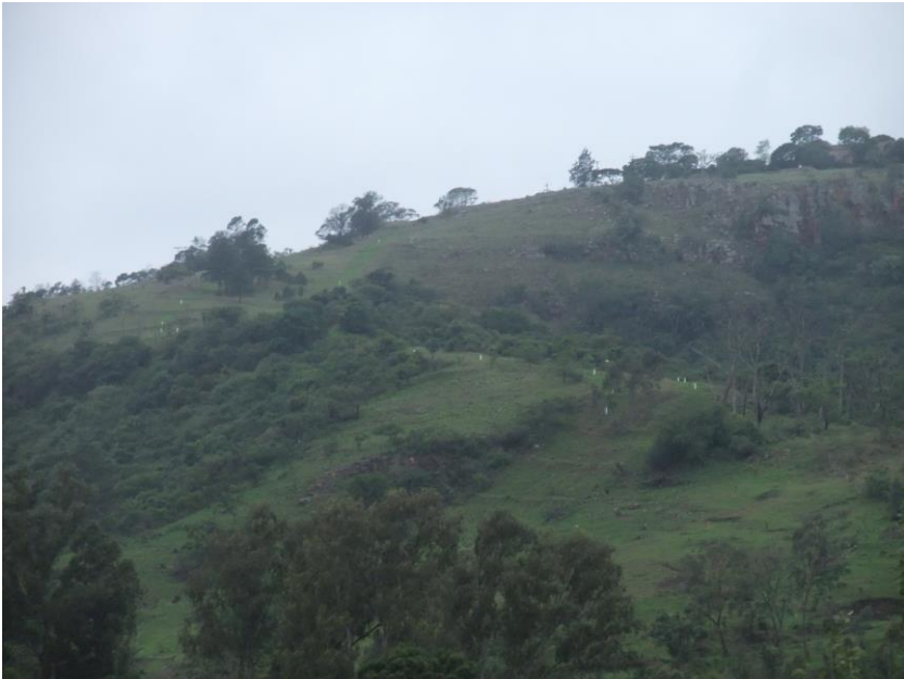
Figure 59: Note the pipeline running across the mountain and through a forestry area.
