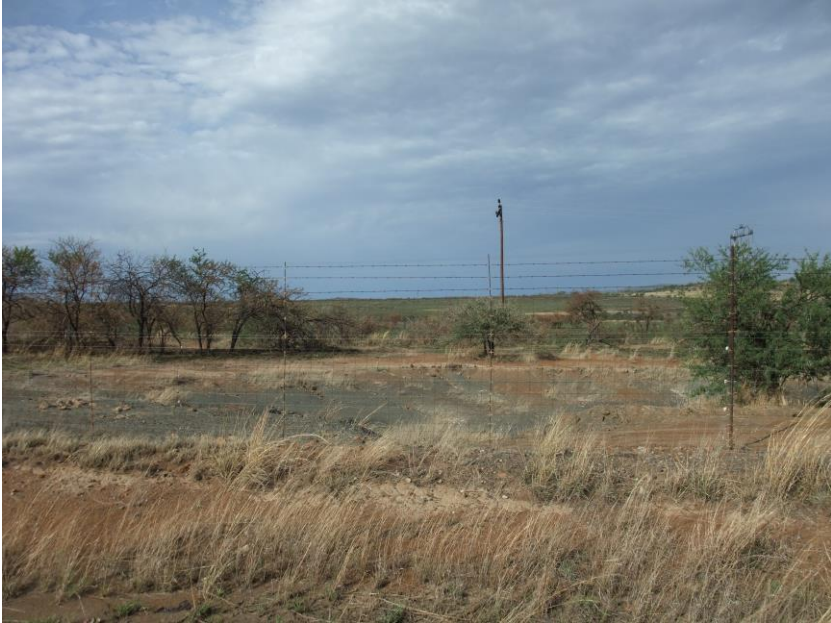
Figure 43: Earthwork activities along the pipeline route.
