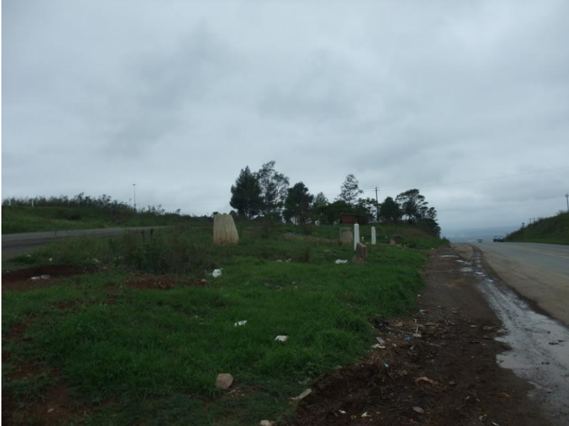
Figure 61: Example of the pipeline adjacent to a road close to a residential suburb.
