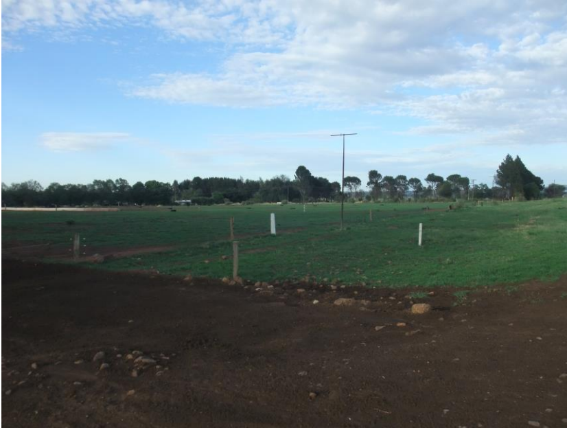
Figure 31: Gravel road along which the pipeline runs.
