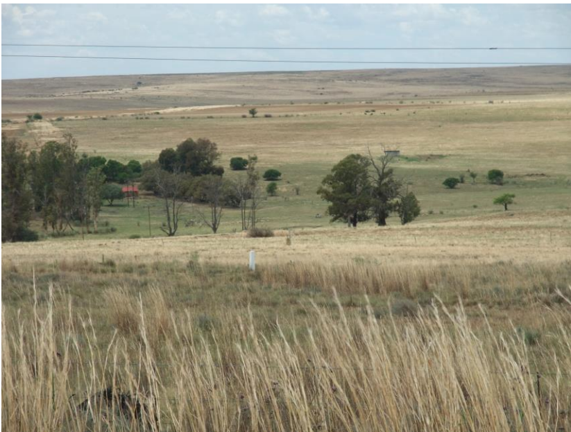
Figure 36: Rolling hills between Kroonstad and Bethlehem where the pipeline runs.
