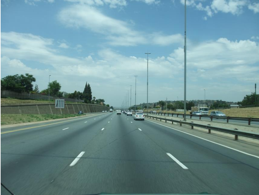
Figure 26: Highway along which the pipeline runs.
