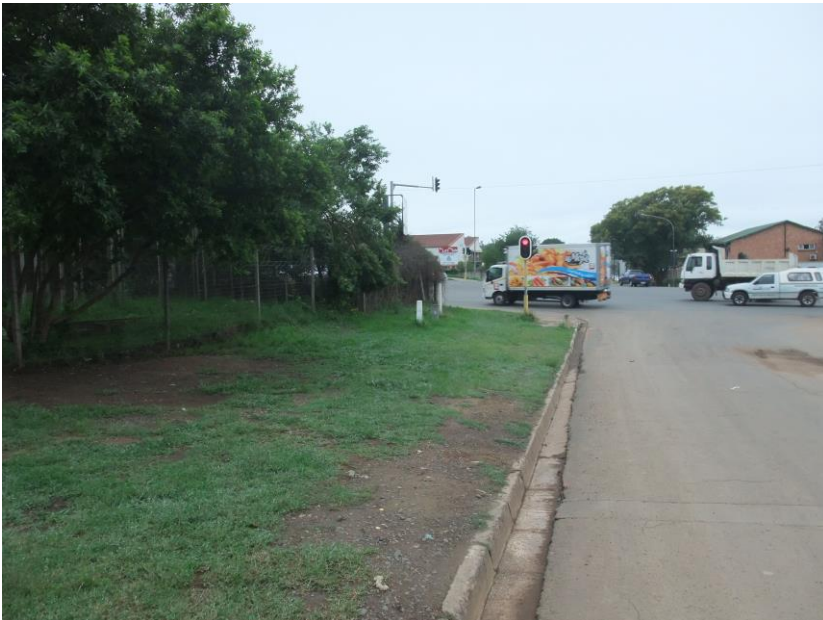
Figure 56: Note the pipeline markers along a street in Pietermaritzburg.
