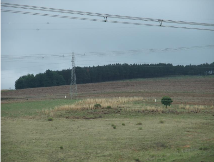
Figure 47: Note the pipeline markers close to a plantation. In some instances it goes through forestry areas.
