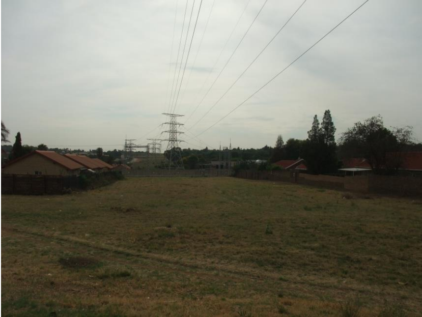
Figure 17: Here the pipeline runs together with power lines.
