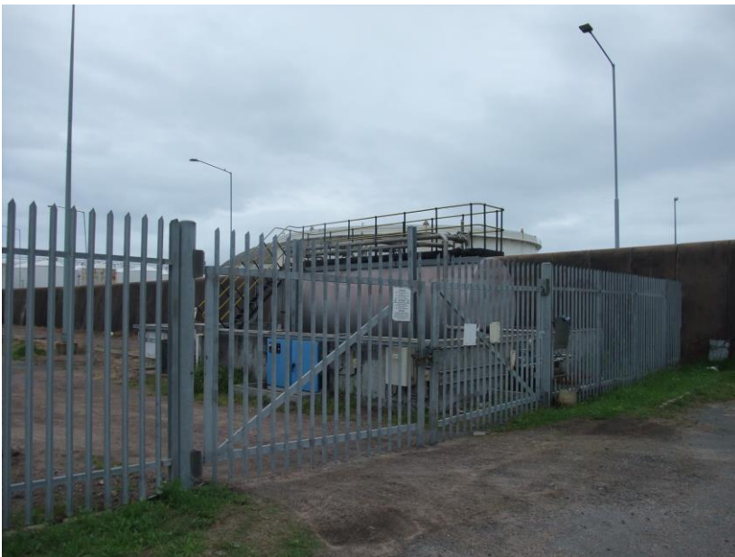
Figure 64: Starting point of the pipeline at the Durban harbour.
