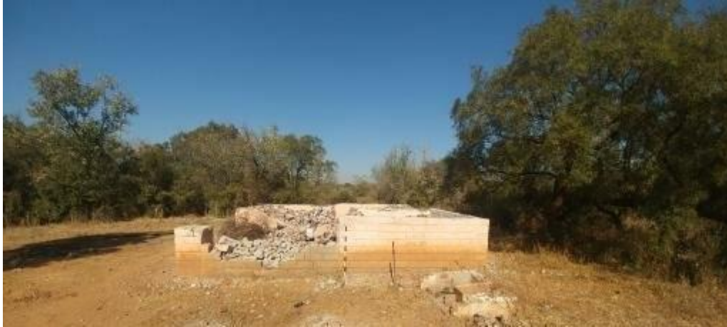
FIGURE 8: REMAINS OF FAIRLY RECENTLY BUILT STRUCTURE ON THE PROPERTY.
