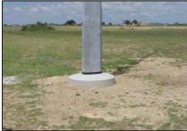
Plate 2: The base of the tower footing.
