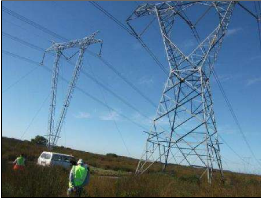
Plate 18: Two existing 400 kV lines and access road.
