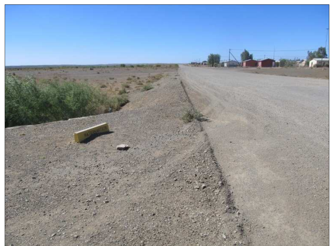
Figure 6. View along Korster Street.
