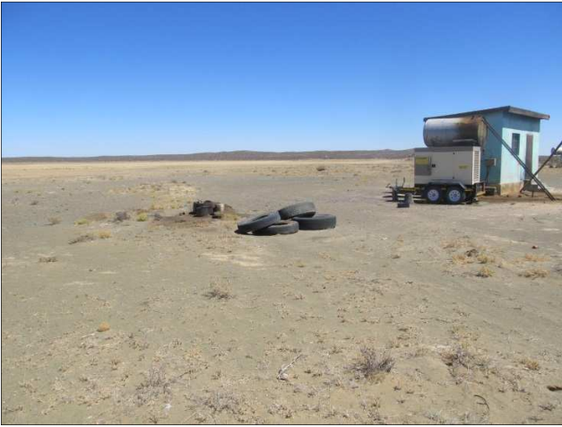
Figure 7. Existing pump station at the unnamed pan.
