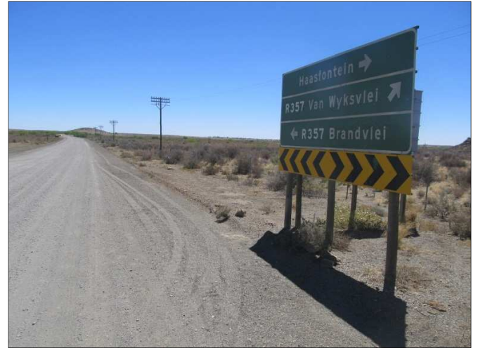
Figure 28. Intersection of R353 & R357.
