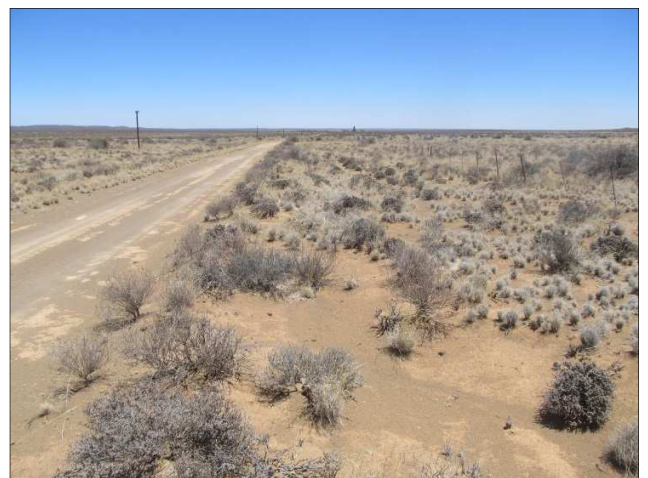
Figure 12. View along OG 86.
