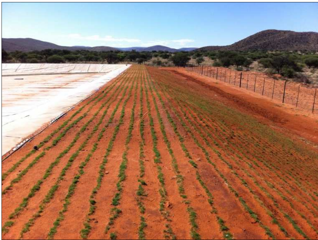
Figure 70. Example of an earth dam in the Northern Cape
