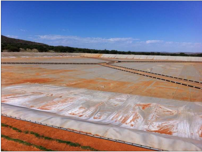
Figure 69. Example of an earth dam in the northern Cape
