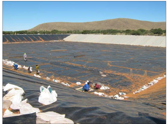
Figure 72. Example of an earth dam in the Northern Cape
