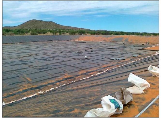
Figure 71. Example of an earth dam in the Northern Cape
