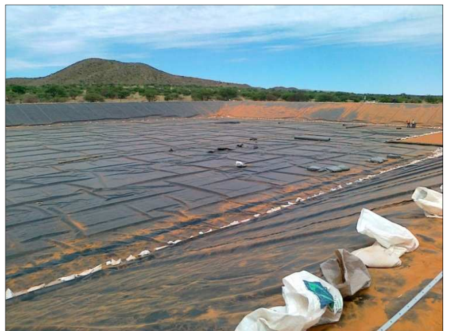
Figure 92. Example of an earth dam in the Northern Cape
