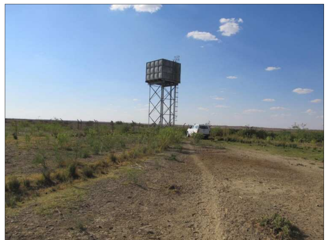
Figure 110. Proposed Loubos pipeline and existing pressure tower
