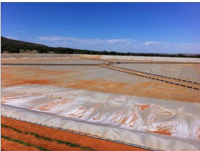
Figure 91. Example of an earth dam in the Northern Cape
