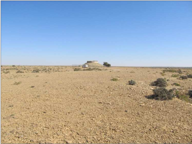
Figure 33. Reservoir at Philandersbron
