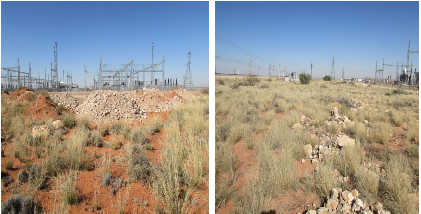
Figure 5: View of section of the proposed area used for dumping/ and storing construction materials.
