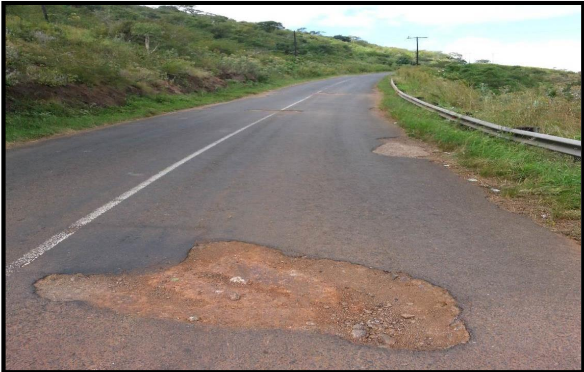
Figure 4. Dense vegetation occurs along the greatest section of the P236.
