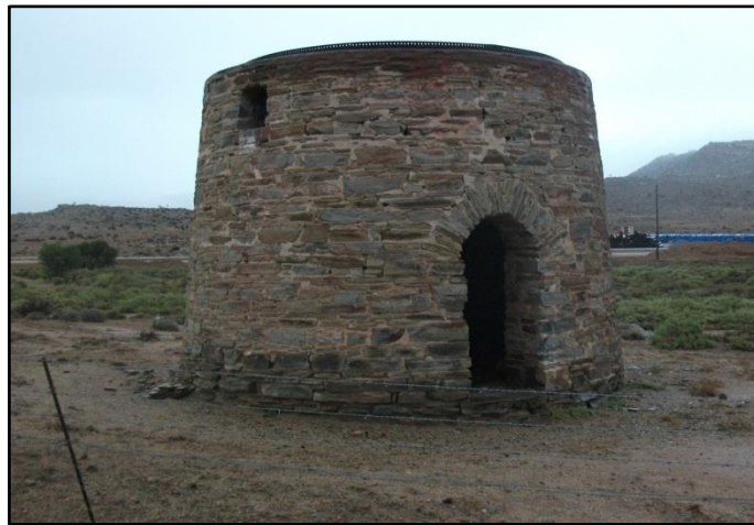
Plate 17: The base of the water tank immediately outside the road reserve.
