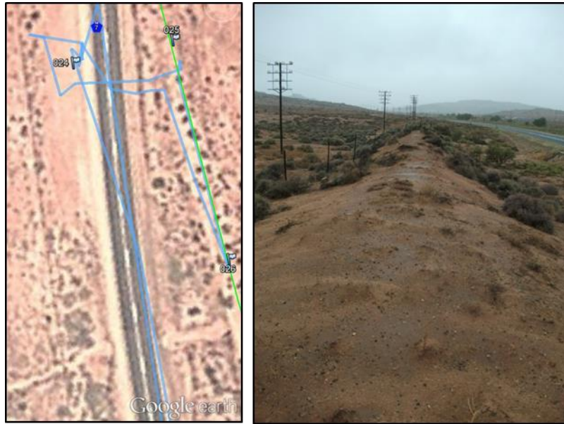
Figure 13: The position of a short section of the railway track between 25 and 26. Plate 13: shows the section of track inside the road reserve, running parallel to the N7. Note the fence on the left.
