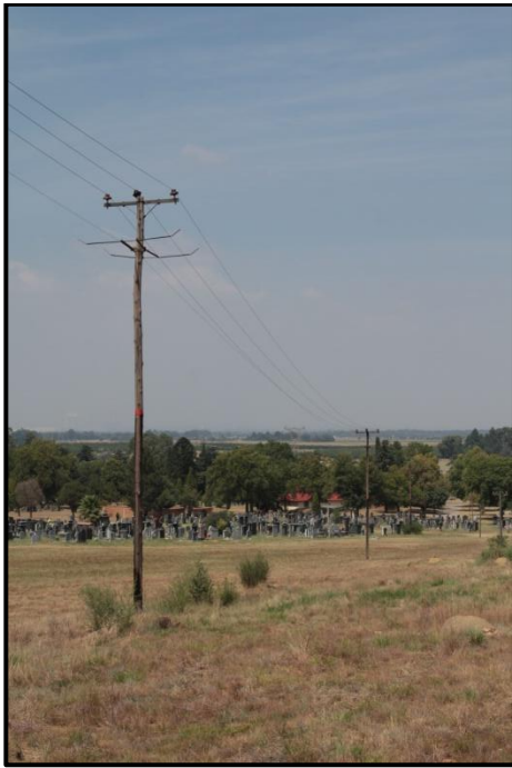
Fig. 6. An existing power line already transects the cemetery and some of the graves.
