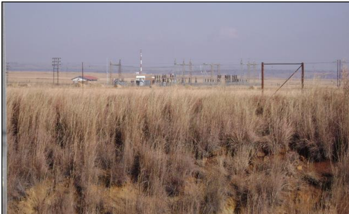
Figure 2: View of the end point of the proposed power line routes at Tweedracht substation.
