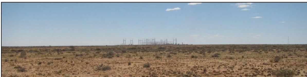
Figure 3: View towards the northeast of the Eskom Nieuwehoop Substation currently under construction at the northern end of the electrical corridor.
