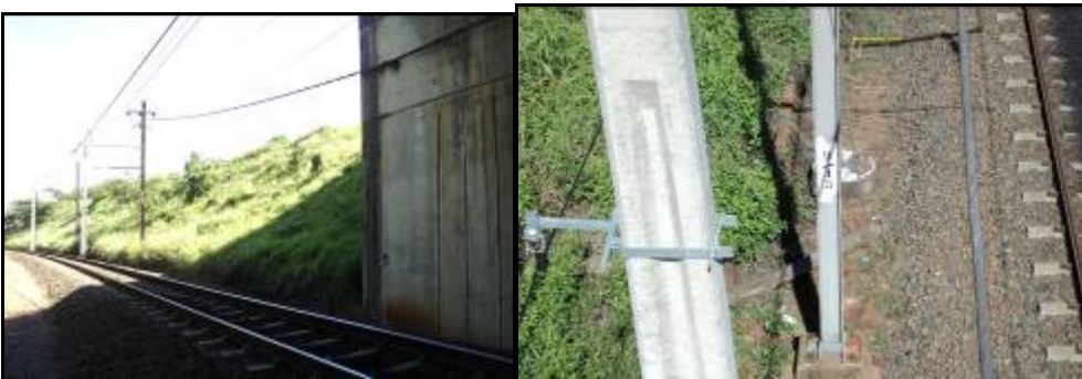
Plate 2: Umhlathuze and Empangeni Rail Bridges
