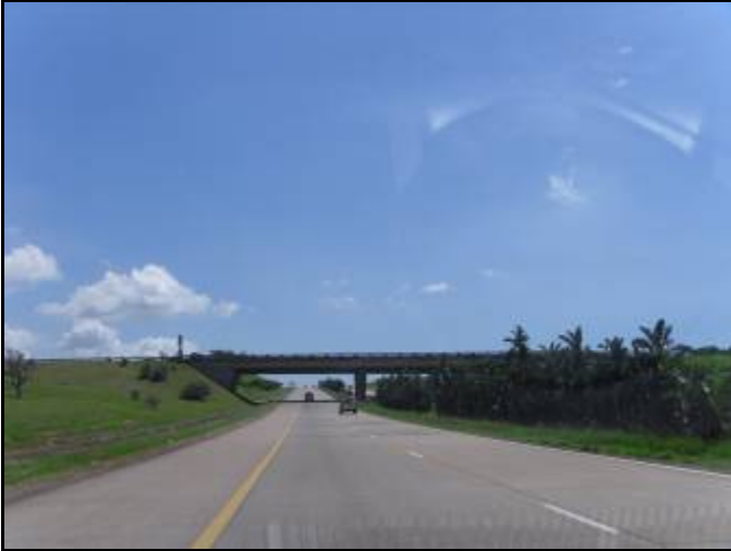
Plate 1: Road currently being used
