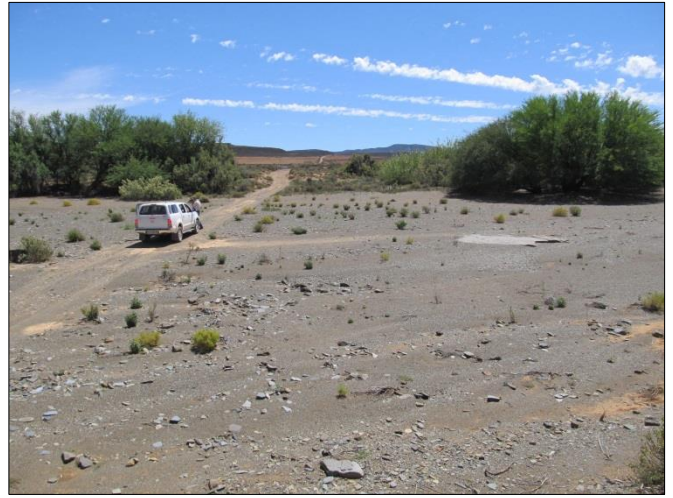
Figure 6 Pipeline route alongside Rheeboksfontein Road
