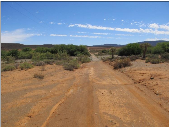
Figure 5. Pipeline route alongside Rheeboksfontein road
