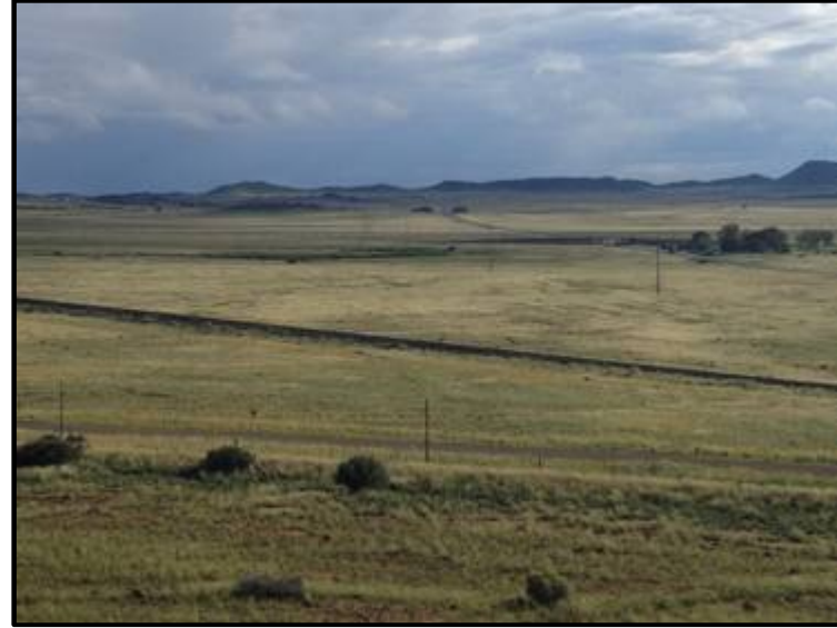
Figure 11. Railway line in the southern portion of the study area.
